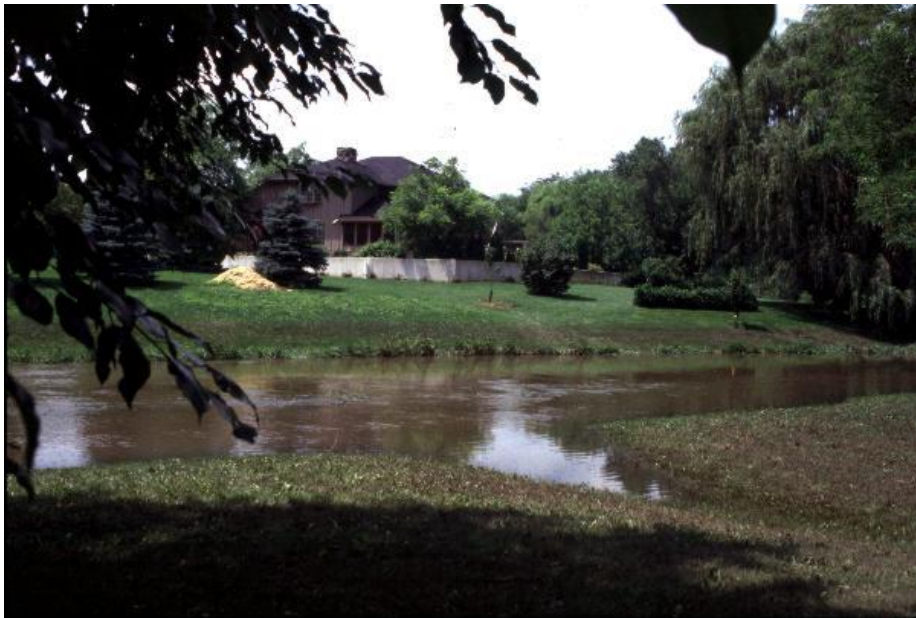
House In Floodplain at Stevens Creek
